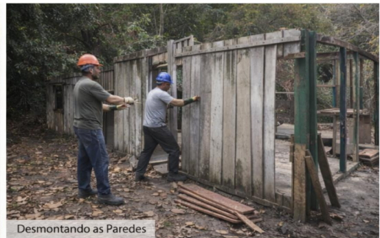
Desmontando as Paredes
